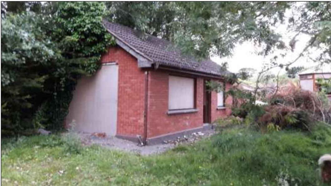
Plate 23. Granny flat in the garden of House 3 in 2018. Up to 5 common pipistrelle and soprano pipistrelle emerged from this building.
