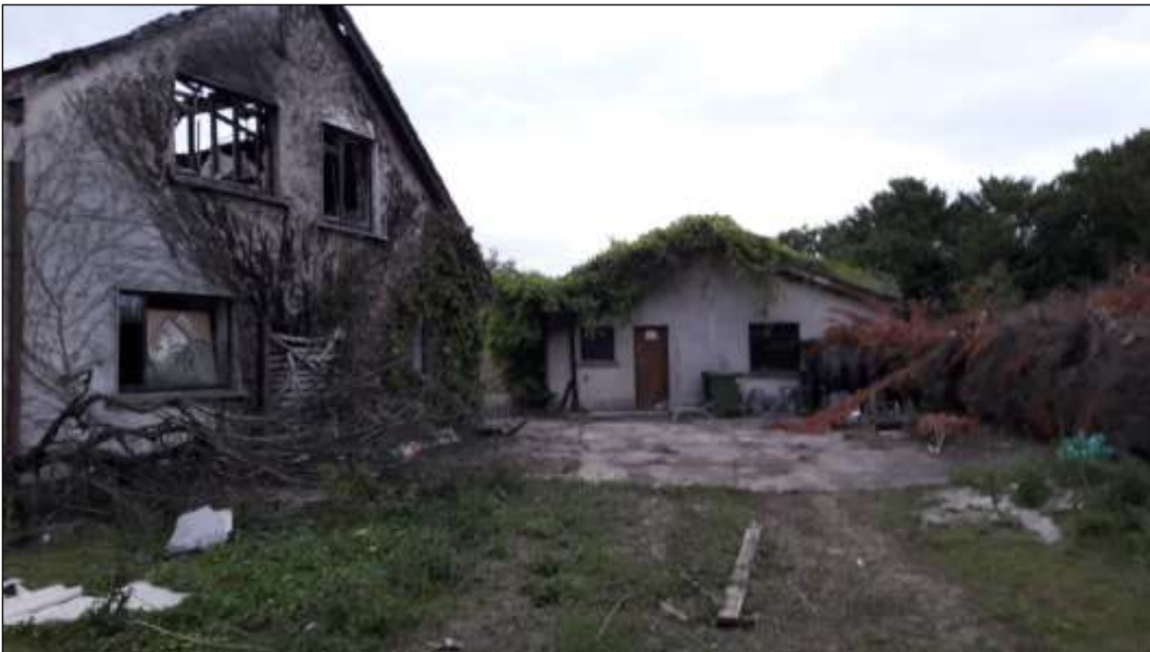
Plate 19. House 2 and detached garage – rear view in 2018.
