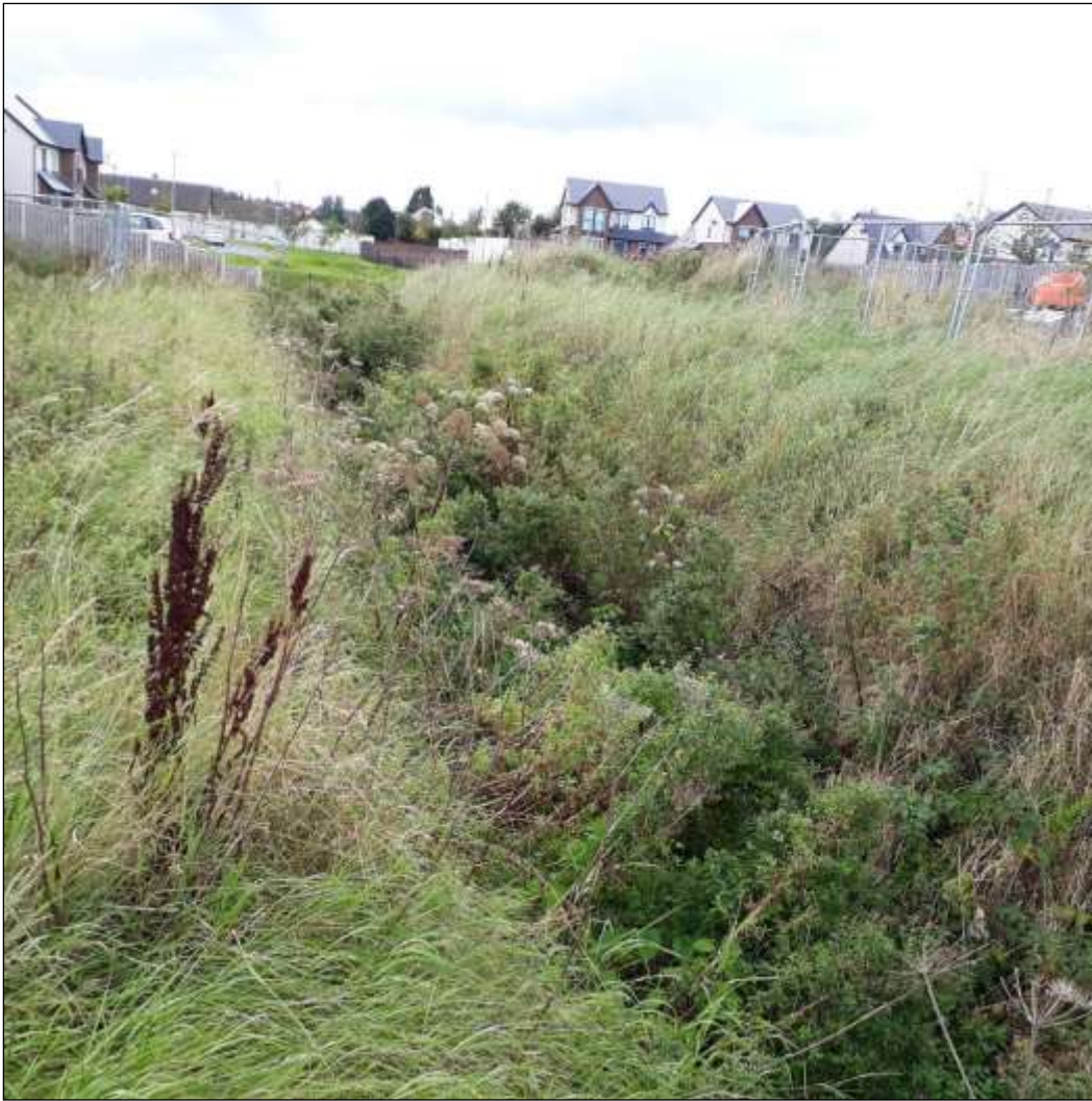
Plate 5. Drainage ditch at the northern boundary of the southern lands.
