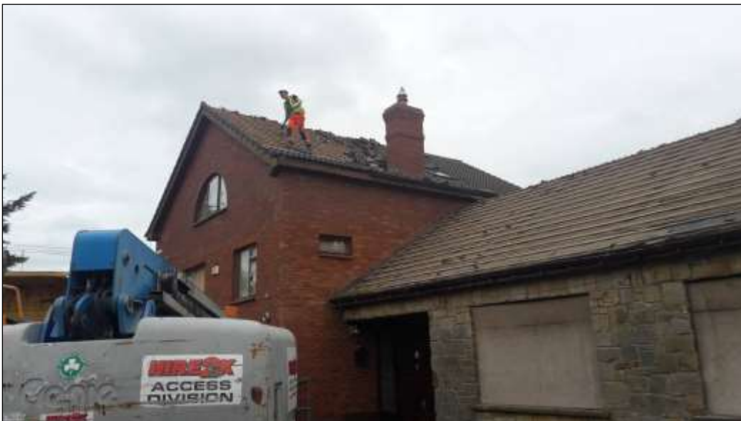
Plate 27. Roof stripping of the easternmost house in October 2018.
