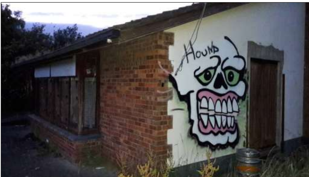
Plate 25. Former rugby clubhouse building in 2018.
