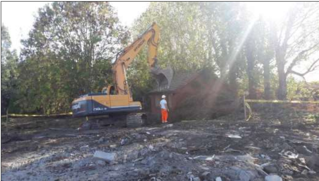
Plate 31. Roof stripping of the granny flat in the grounds of the easternmost house in October 2018.
