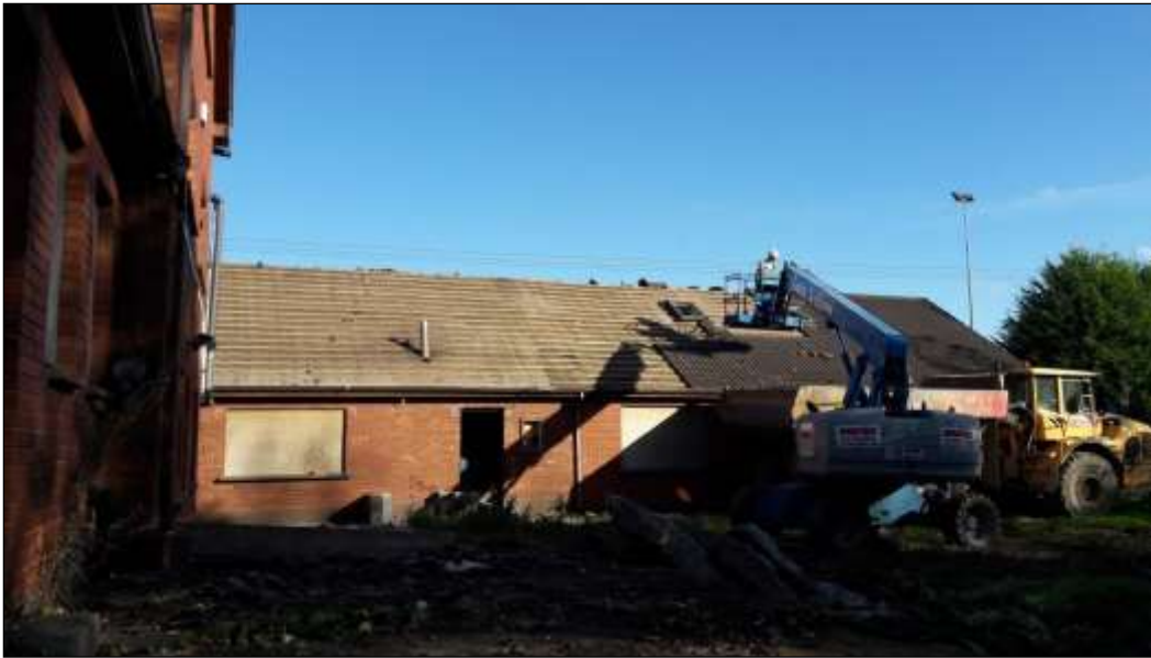
Plate 28. Roof stripping of the easternmost house in October 2018.
