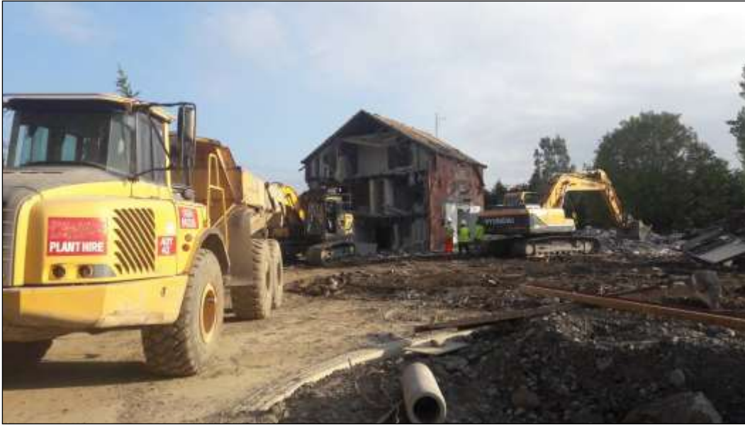
Plate 30. Demolition of the easternmost house in October 2018.
